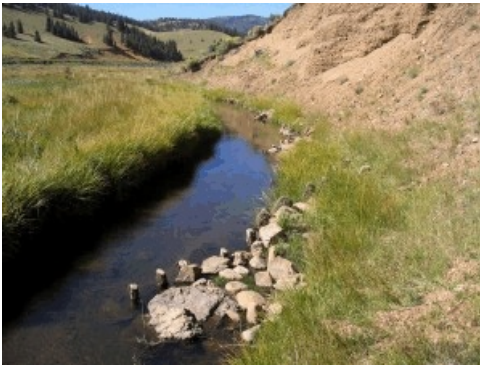
Post vanes installed along Comanche Creek - note sedges and grasses re-establishing along raw right bank.
